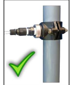
7. Establish the pipe diameter you have installed and make sure you have the correct pipe saddle (50 or 63mm).
