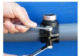
12. Wrap the threads of the saddle fitting adapter ( $\frac{1}{2}$  to  $\frac{3}{8}$ ) with Teflon tape and thread it into the acid pipe saddle.
