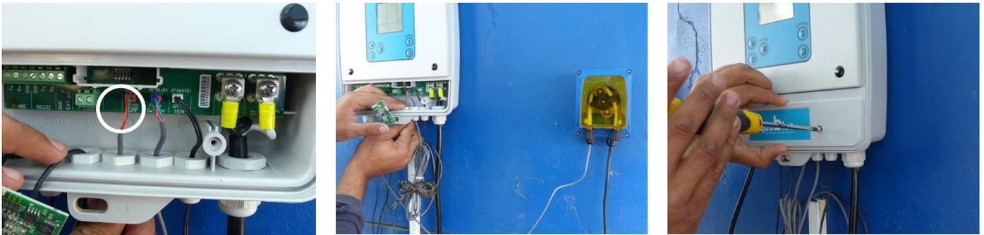
Wire the electrical cable of the acid pump to the main power source in the machine room (240V) parallel to the circulation pump. **This must be performed by a licensed electrician!**
